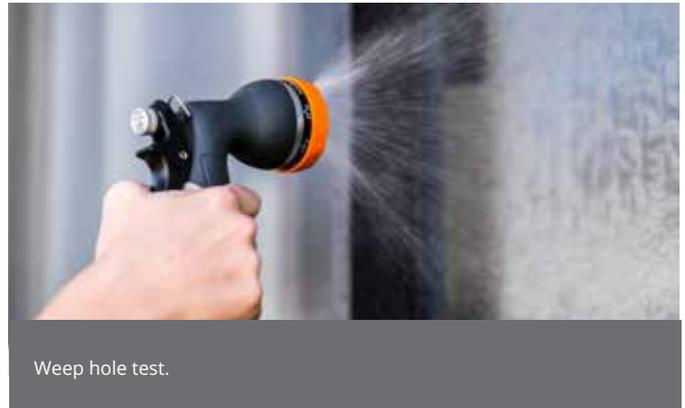
A good method to test your weep holes for adequate drainage is to run your hose over your windows or sliding door, checking your weep holes are letting the water flow out freely and not overflowing. Use a fine spray on your hose from a distance of 2 metres rather than a full blast when performing this test.
